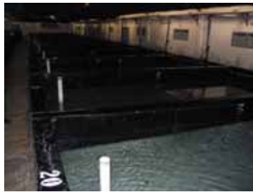
Figures 10 & 11: Epoxy painted larval rearing tanks
