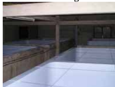
Figures 10 & 11: Epoxy painted larval rearing tanks
