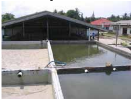
Figure 4: Gravity sand filter
