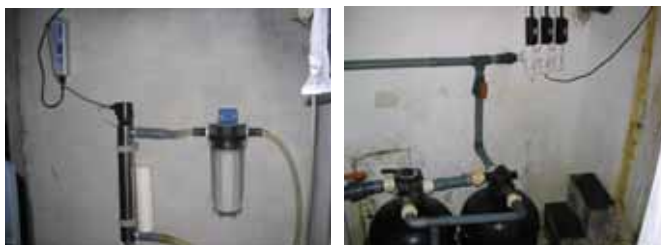
Figures 22 & 23: Cartridge and UV filtration systems for spawning/hatching tanks
