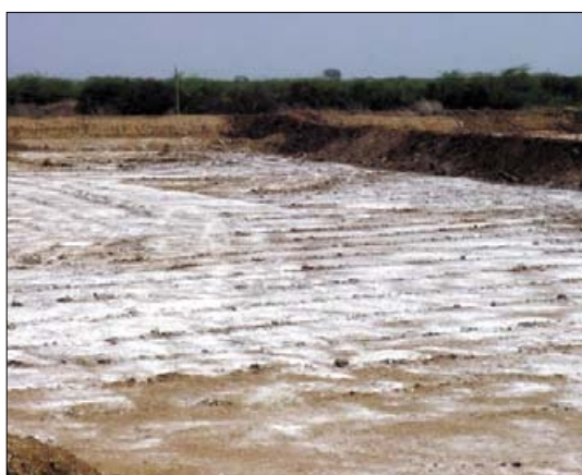
Lime application to pond bottom
