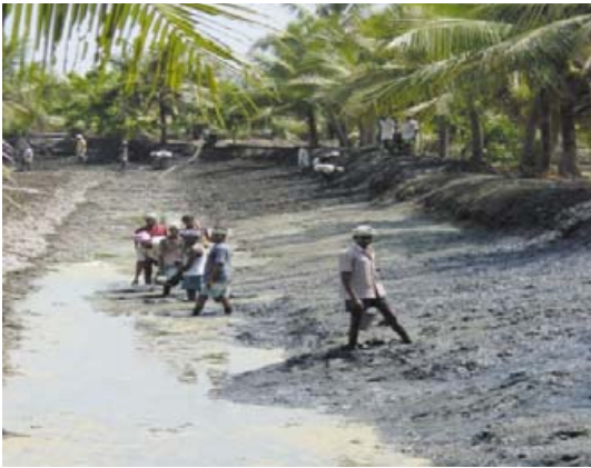
Manual removal of sludge
