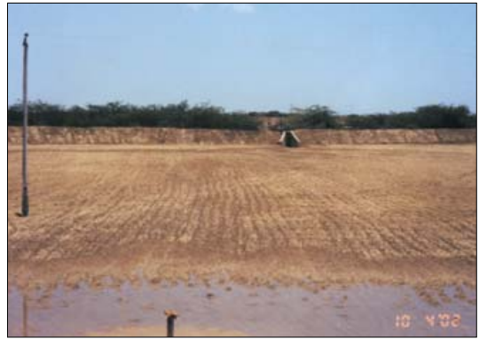
Ploughing on dry soil and subsequent wetting of bottom
