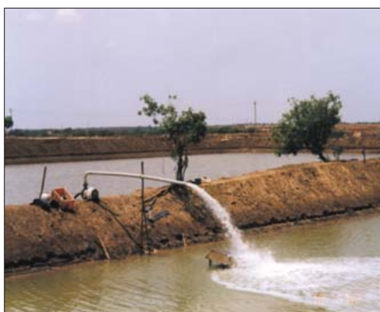
Clean water pumped from the reservoir pond
