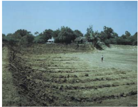
Mechanical sludge removal using bulldozers
