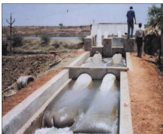
Water filtration by twin bag filter (Nellore district)
